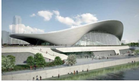
Figura 19: Zaha Hadid, 2005 – 2011, London Aquatics Centre, London, UK. Fonte: Lomholt, Isabelle, 'London Aquatics Centre: Olympics Swimming Venue', in London Aquatics Centre: Olympics Pool by Zaha Hadid (e-architect, 3 aprile 2016)
